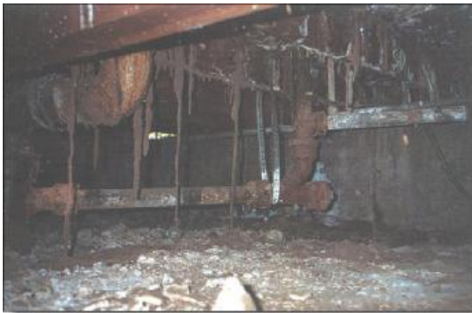
Entrance to crawlspace # 3
